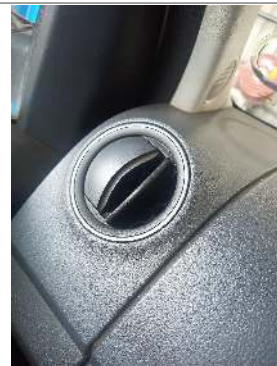
Central Air Vent
