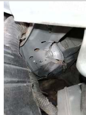
Main Beam Left
