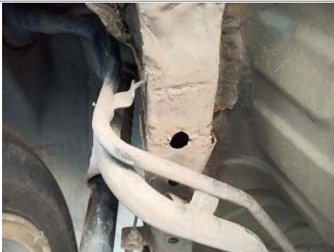
Main Beam Left
