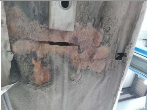
Floor pan cut
