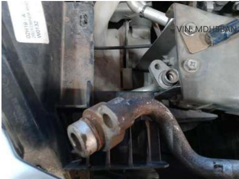
Air conditioner pipes
