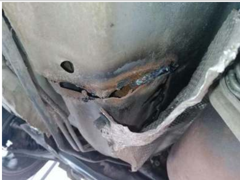
Floor pan cut.
