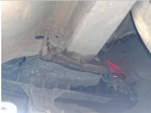
Main Beam Left
