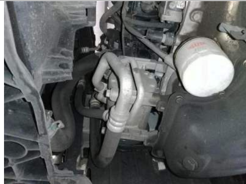
Air conditioner pipes
