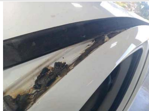
Channel / Roof Gutter Left
