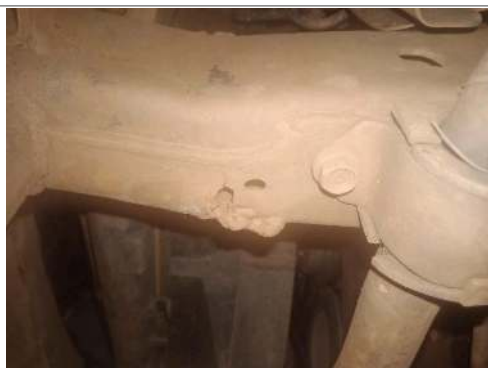
Main Beam Left
